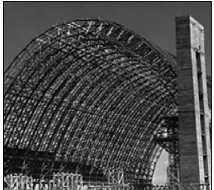
Fig. 8: The catenary arches under construction 49
