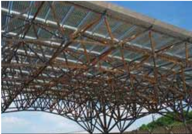
Fig. 15: Solar canopy at The Earth Centre, larch space frame construction
