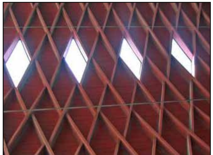
Fig. 10: Lamella barrel roof at Hounslow East Station
