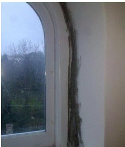
1. Window reveal showing black mould caused by condensation on cold surface
