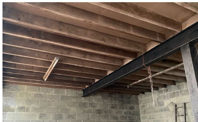
Figure 4: Farm infrastructure constructed using on-farm timber. Images by Anna Dauksta.
