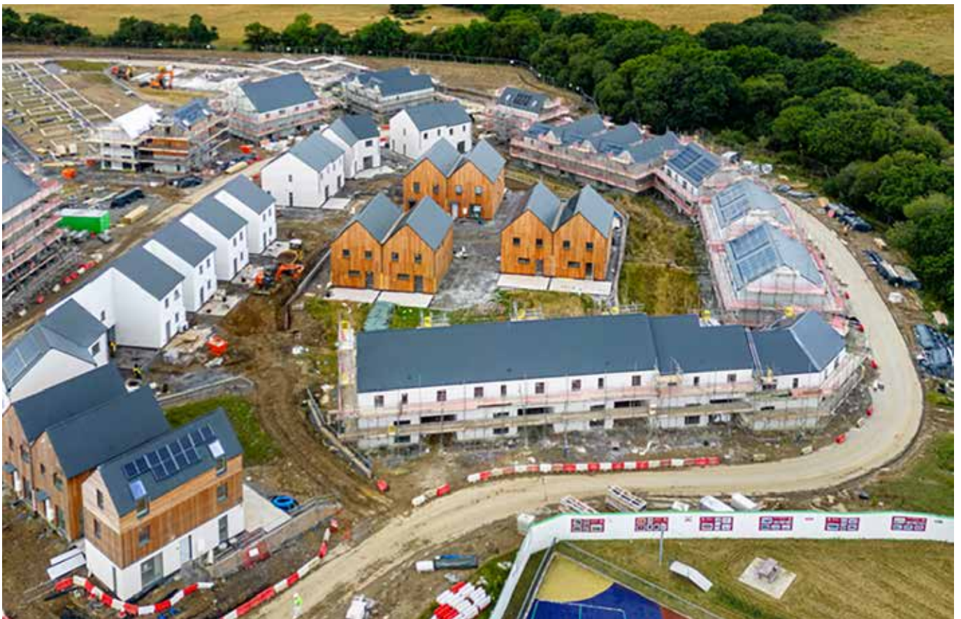
Part of the site under construction (© Buffoon Media)
