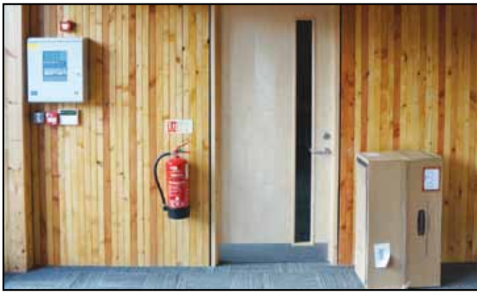
Figure 31: Interior of Coed y Brenin extension showing Dowellam wall
