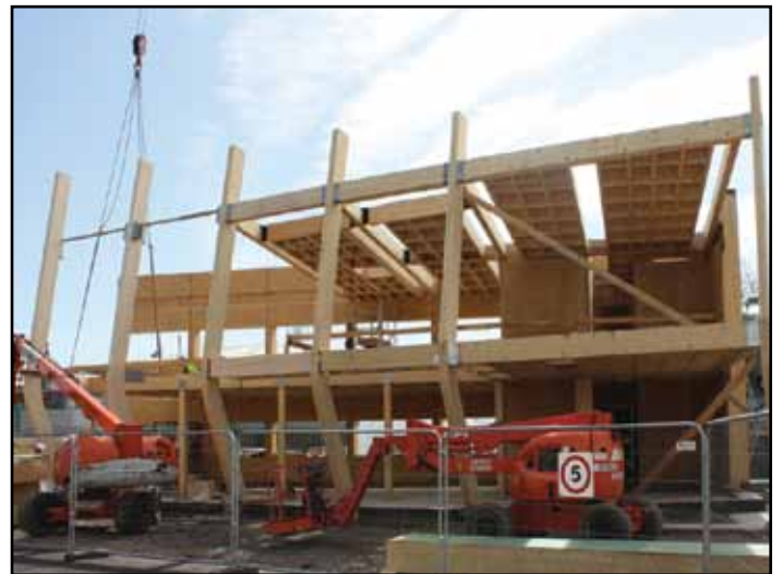
Figure 6: Treglown Court glulam structure being erected (image: courtesy of Stride Treglown)
