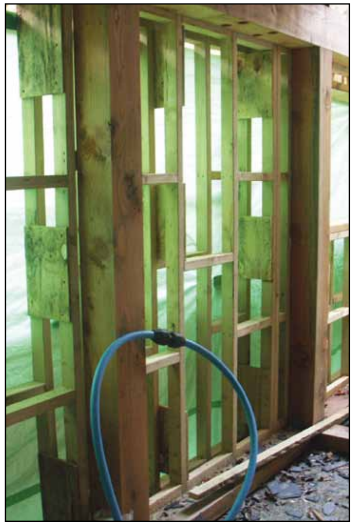
Figure 8: Local Douglas fir post and beam structure with low thermal bridging twin-wall envelope
