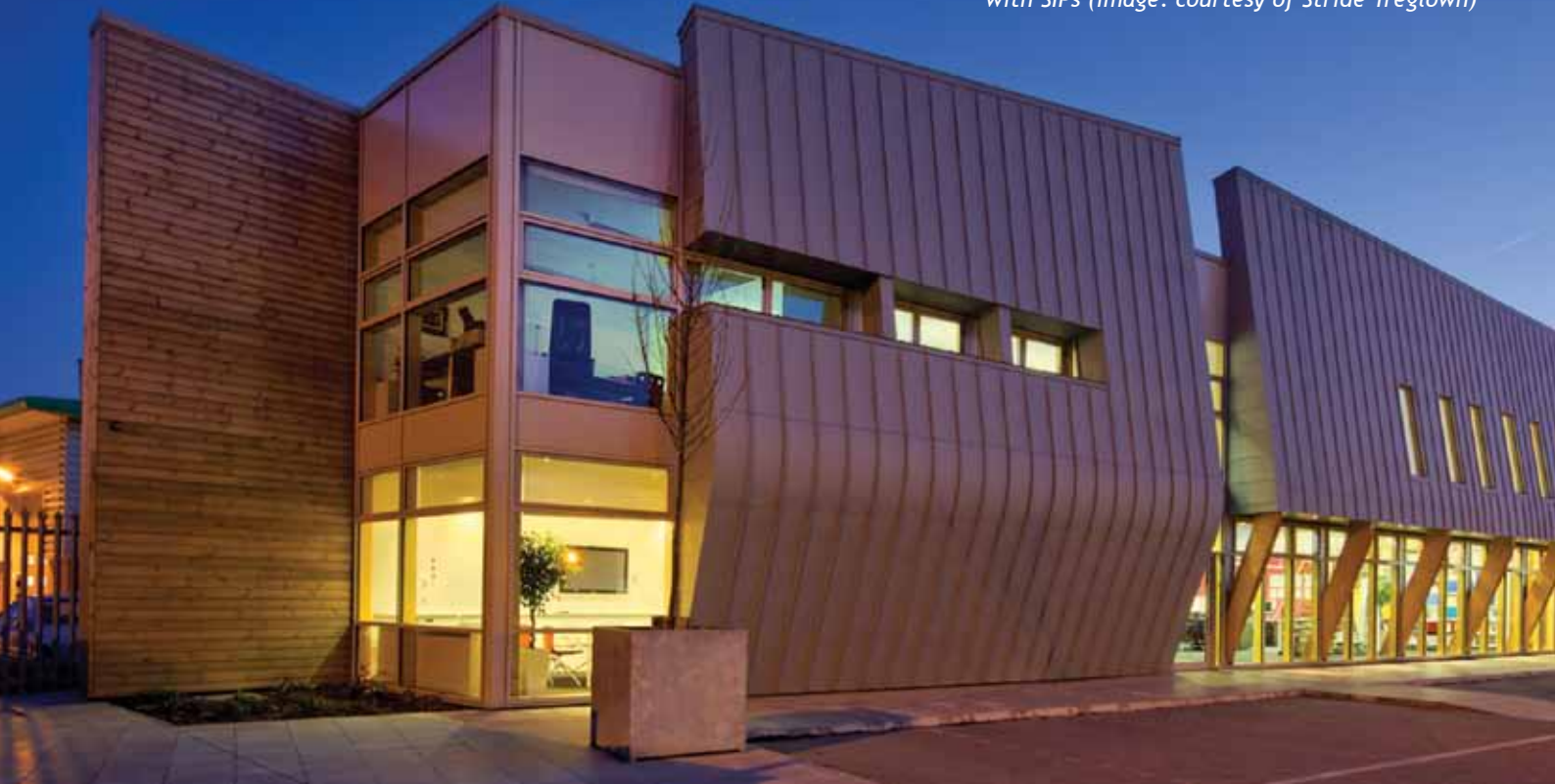
Figure 5: Treglown Court in Cardiff, glulam post and beam with SIPs (image: courtesy of Stride Treglown)
