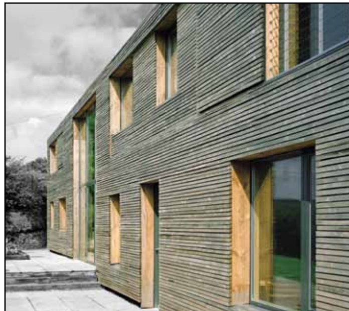
Figure 28: Ty Pren 'longhouse' uses SIPs with larch cladding (image: courtesy of D. Grandorge, Feilden Fowles)
