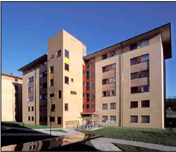
Figure 14: Six storey open panel student housing at Swansea University (image: courtesy of Architype)
