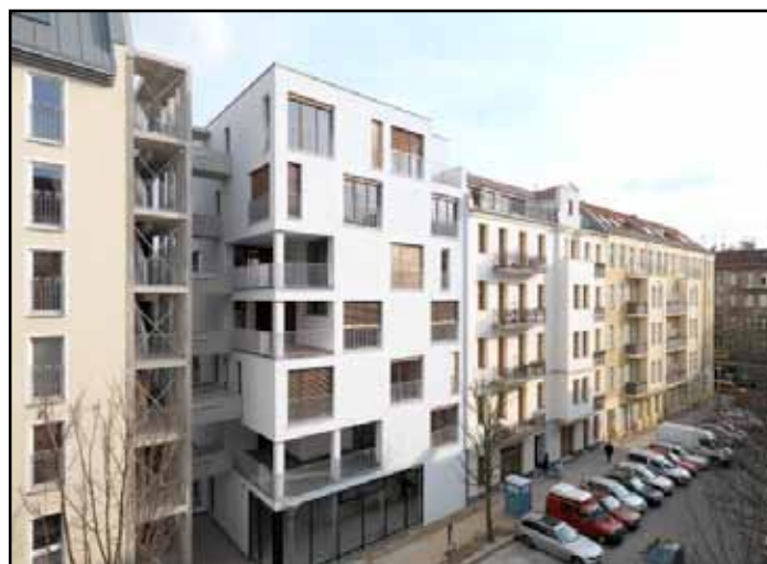
Figure 30: The seven storey Brettstapel e3 apartment block in Berlin (image: courtesy of Bernd Borchardt and Kaden + Klingbeil)
