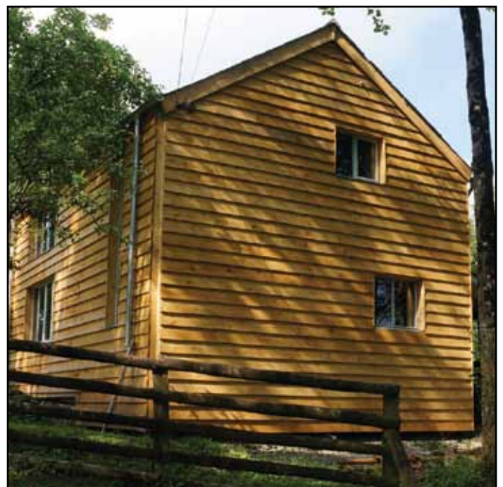
Figure 4: Homegrown western red cedar cladding on a house in Mid Wales
