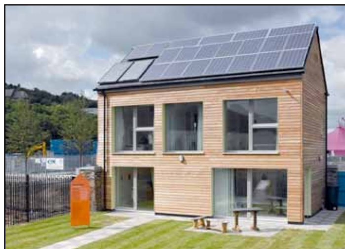
Figure 22: Larch House in Ebbw Vale used closed panel construction and larch cladding
